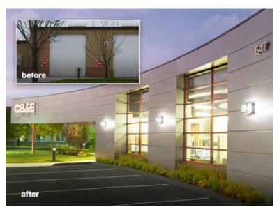
A utilitarian former state vehicle emission testing building just outside of St. Louis, Missouri has been transformed into an eye-catching office building thanks to the remarkable ability of Dryvit's new Reflectit finish to replicate the look of metal panels at a budget-friendly cost.
