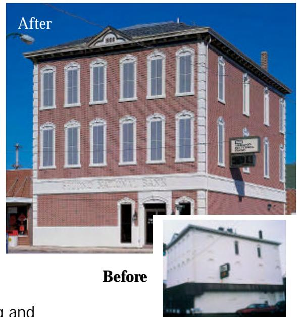
All in all, 5,300 square feet of Dryvit and Custom Brick finish were used to complete the job. The system was installed directly over the existing painted masonry using standard adhesive in combination with mechanical fasteners.
