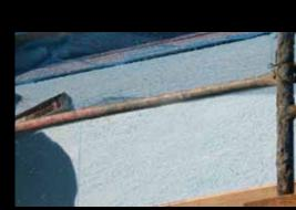
After installation, the surface of DOW™ XNERGY™ insulation is rasped to create a level surface for the application of base coat, mesh and finish layers.
