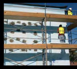
An adhesive/drainage medium is applied to the surface of DOW™ XNERGY™ insulation boards, which come planed for optimal adhesion.
