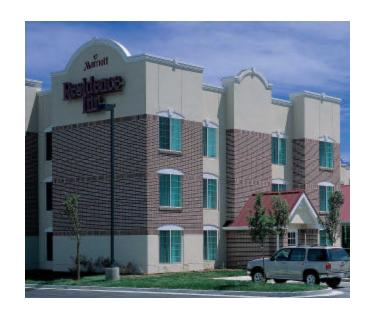
Brick finish to existing brick used in the surrounding area. To do this, Dryvit obtained samples of the 'local' brick, which contains black and white flecks, and duplicated this effect by adding colored quartz aggregate to the Custom Brick finish. Next, a template pattern was selected which matched the original design for the brick itself.
